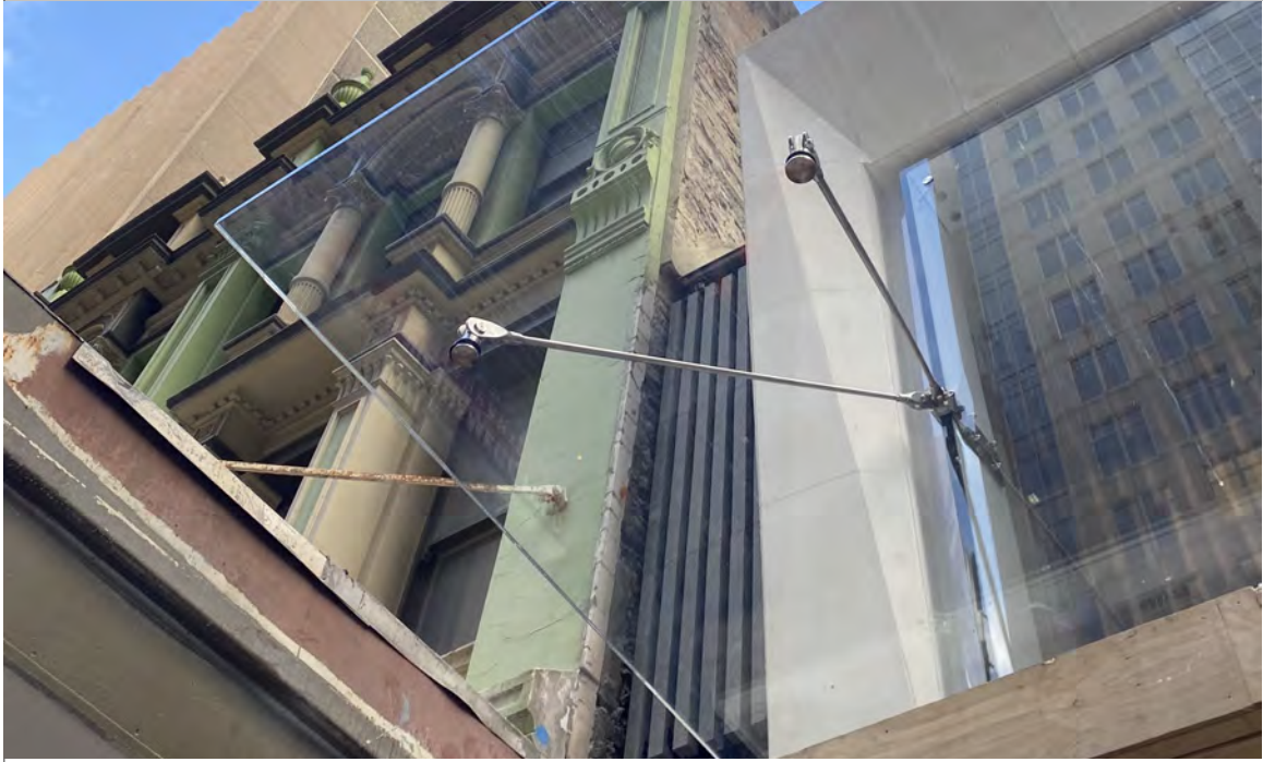
Photo 7: Looking from the ground towards 15 Hunter Street
